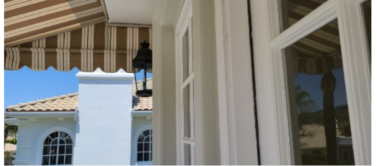
Some lights do not turn on. They may be connected to solar sensors and only come on at night
