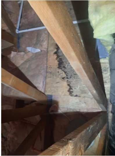
Staining on the floor near the rear furnace.
