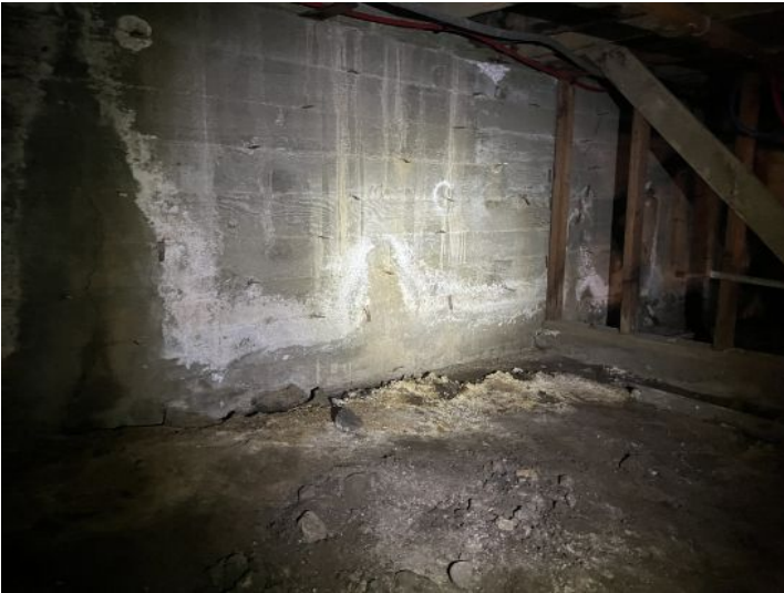
Efflorescence
