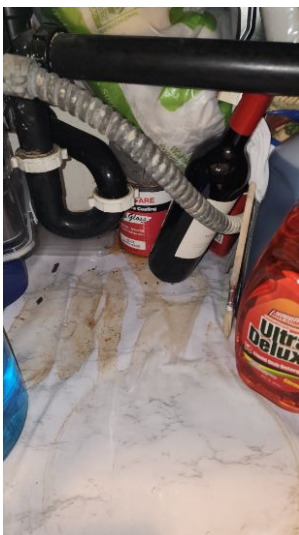
Drain leaks
