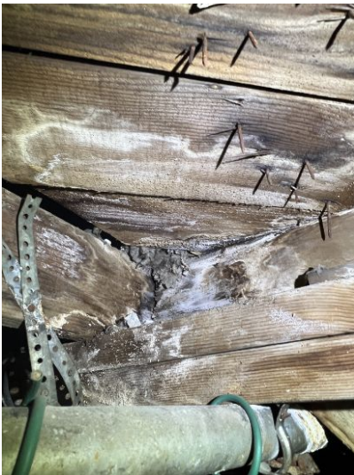
Staining & deteriorated
