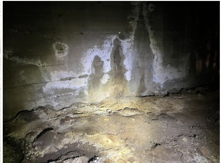
Efflorescence
