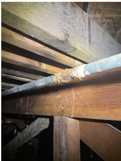
Corroded
