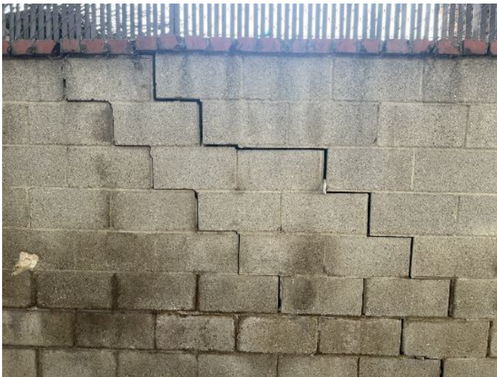
Step cracking
