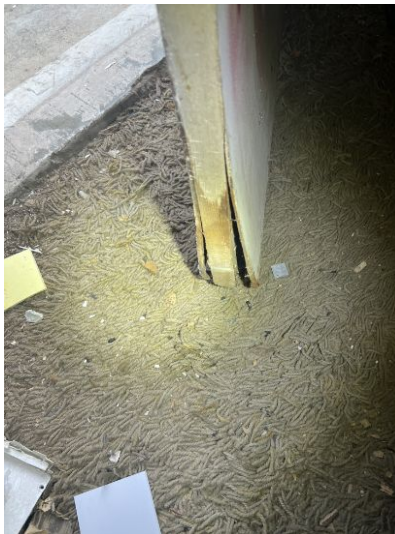
Door to the crawl space
